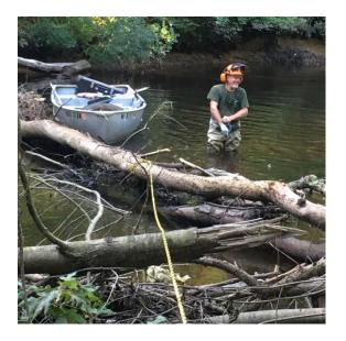
Following the evaluation, the team selectively trimmed, sawed, hoisted, and otherwise cleared enough wood to allow a passageway 6 feet wide with at least one foot of water through fifteen woody obstacles. The removed wood was then relocated back into the channel nearby to preserve the ecological values of instream wood. The result was safer and easier canoe passage through this section with no loss of instream wildlife habitat and no significant changes to natural hydrology.
