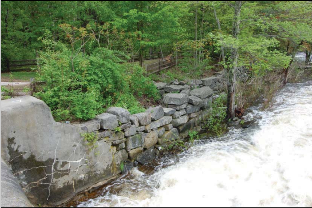
Photograph 3. Structure 2 – Sawmill Foundation, west/center wall, view southeast.
