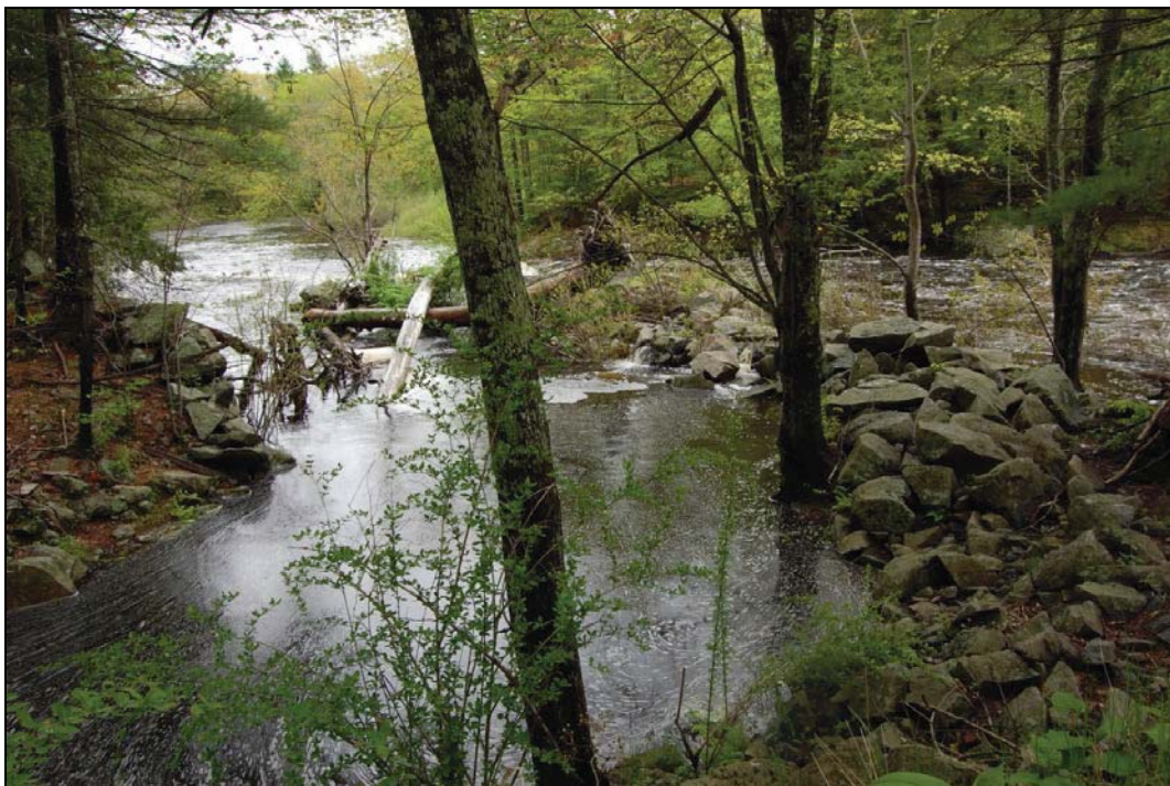
Photograph 2. Rip-rap breakwater at Power Canal outlet, view southwest.
