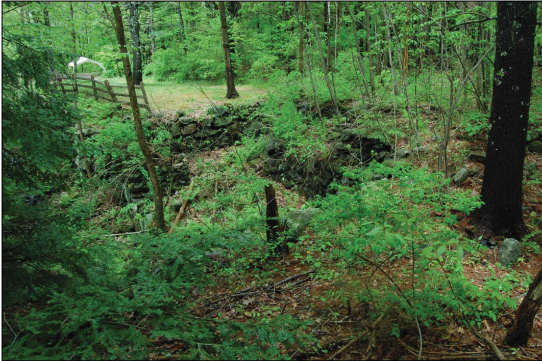
Photograph 7. Structure 3- Paper Mill Foundation, southeast corner, view northeast.
