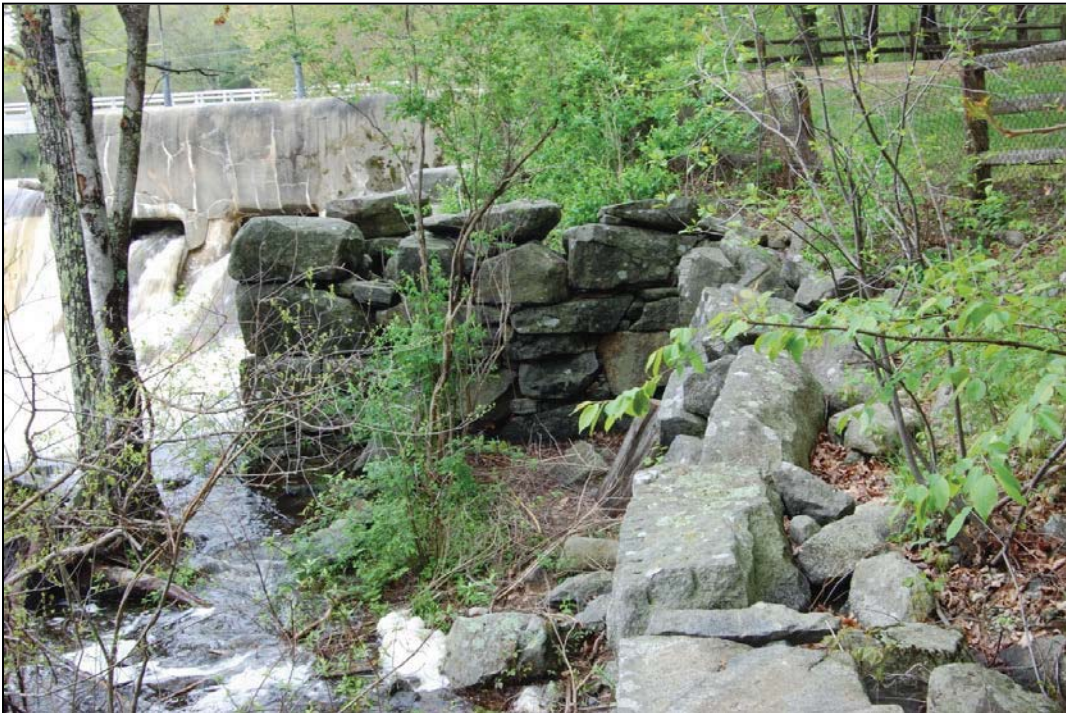
Photograph 4. Structure 2 – Sawmill Foundation, south wall, view north.
