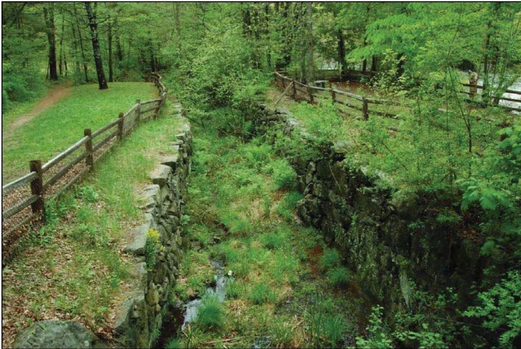
Photograph 1. Structure 1 – Power Canal, view south.
