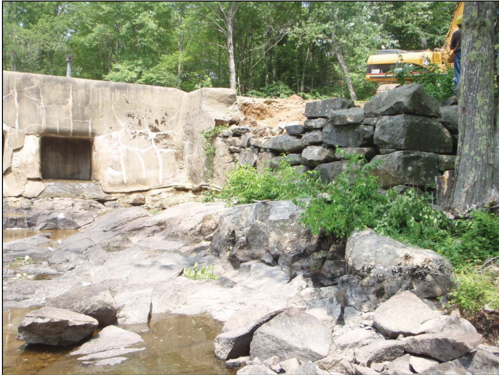
Photograph 6. Possible former exterior foundation/raceway wall of Structure 2 – Sawmill Foundation, view northeast.
