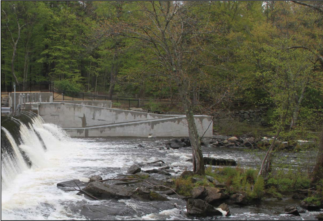
Photograph 5. Reconstructed fish ladder with corner of the Sawmill Foundation preserved in place, view east.
