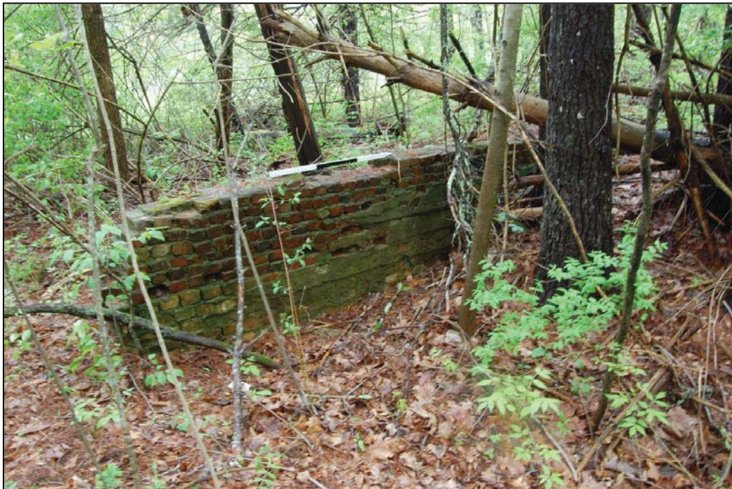
Photograph 10. Structure 4 – Boiler Room, southwest brick foundation wall, view northeast.
