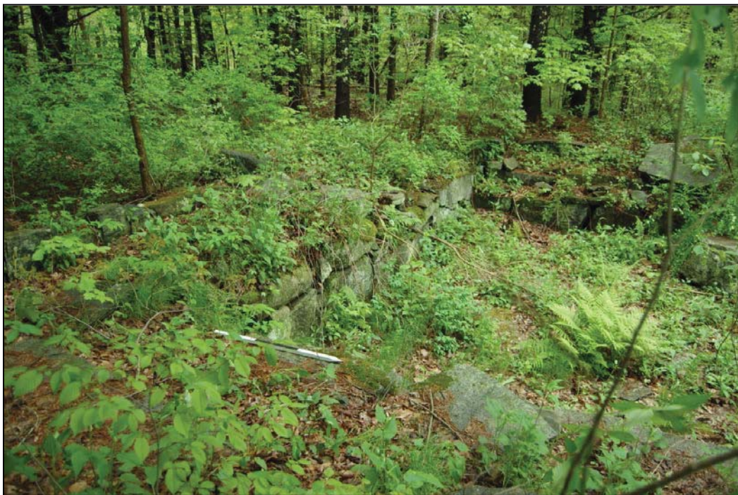
Photograph 12. Structure 6 – Bridge Retaining Wall, view southeast.
