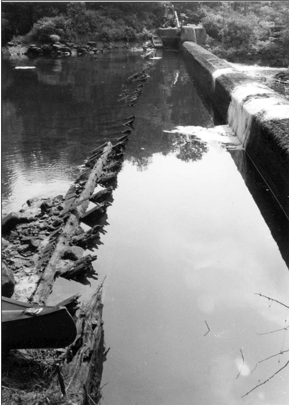
Photograph 16. Structure 11 – 1868 Crib Dam Remains, view east.
