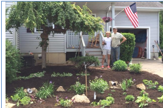
The Great Bay Stewards used their Small Grant to excavate a site being used for a rain garden demonstration project in Newmarket.
