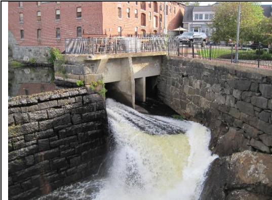
North side: The old flood gate during pre-construction draw-down. Sept. 1, 2020
