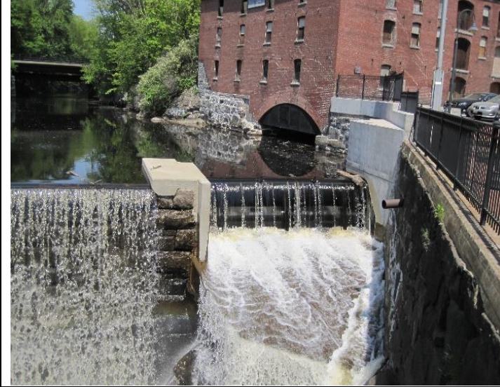
The new flood gate at Macallen Dam.
