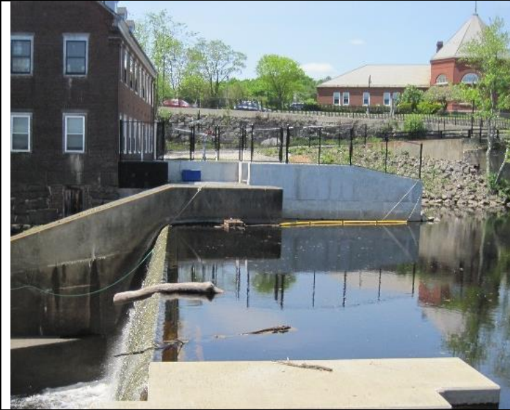
South wall of Macallen Dam after repairs.
